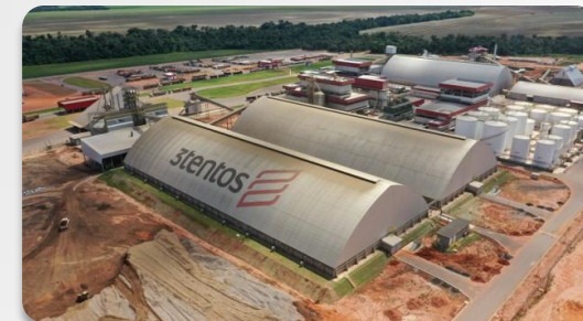
Soybean Processing Plant (Mato Grosso)
