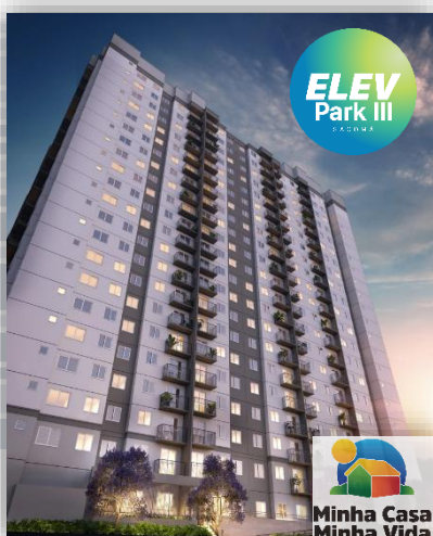
*3D facade of Elev Park Sacomã.
