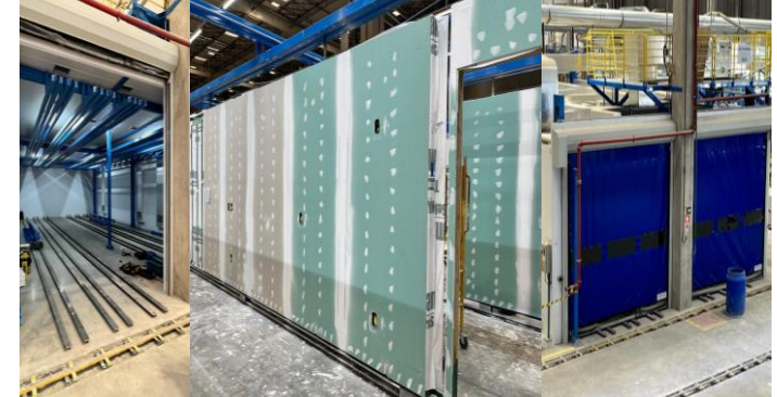
3. Panel caulking station and drying chamber
