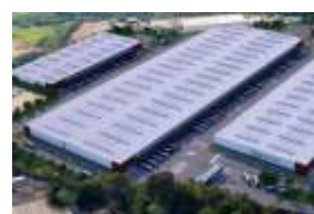
CLD (under construction) Warehouse São Paulo / 2023 128,516 sqm - total (17.03% SYN) 74,139 sqm - delivered
