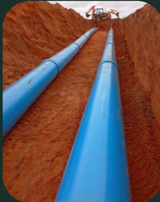
Water Main Installation 500mm
