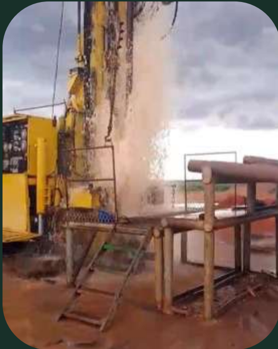
Well drilling 300m 3
