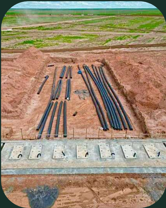
Construction of the pump house
