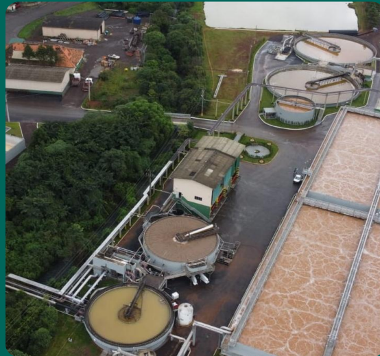
EFFLUENT TREATMENT PLANT CDM
