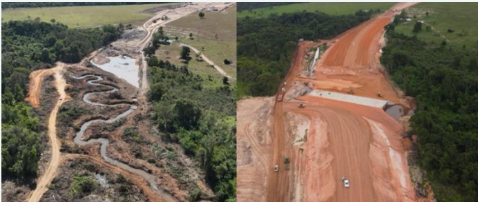
Earthworks in critical sections (km 56)
