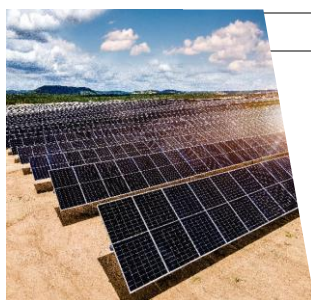
PHOTO: Luzia Solar Complex - PB
