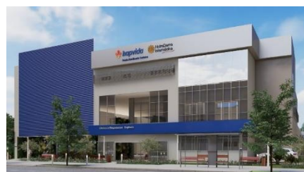
Contorno New Emergency unit – Belo Horizonte/MG – apr'23
