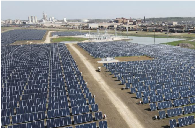
Solar Panels & Midlothian Industrial Unit
