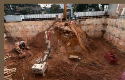
Excavation and ground anchors
