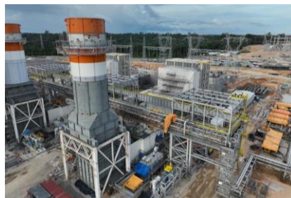
UTE: Flushing do lube oil
