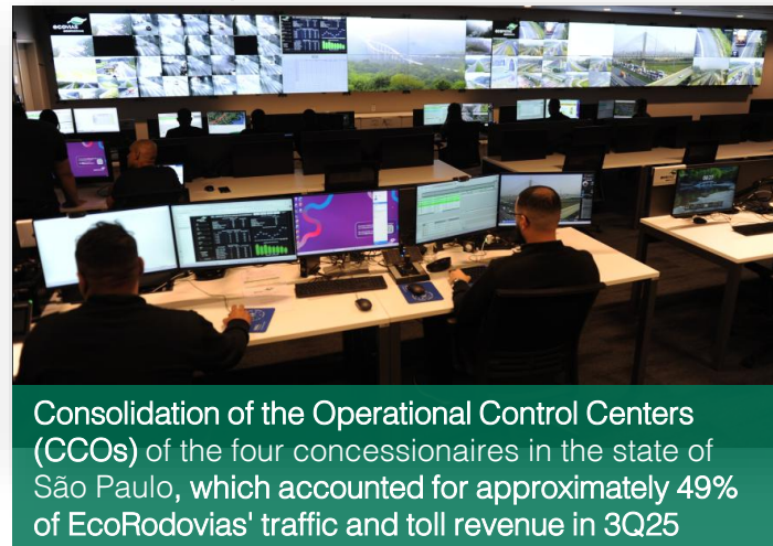
São Paulo Operations Center
