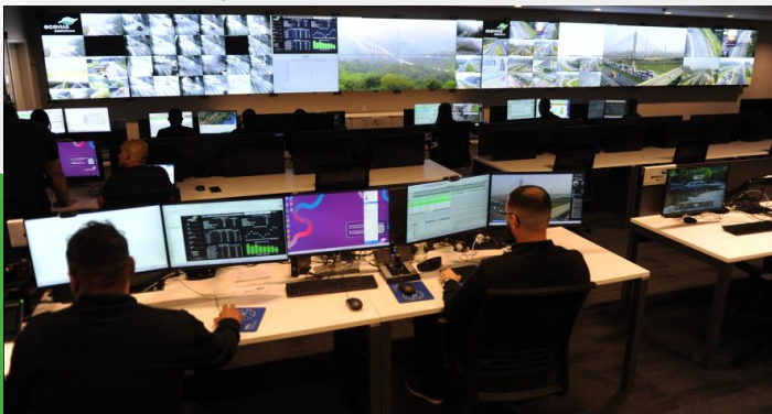
São Paulo Operations Center
