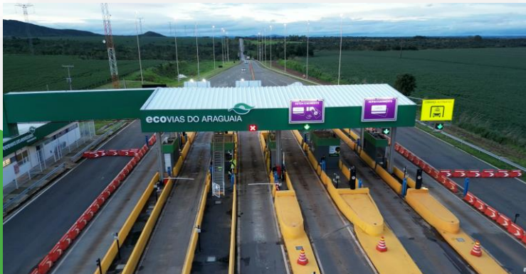
Autonomous toll plaza | Ecovias Araguaia and Rio Minas
