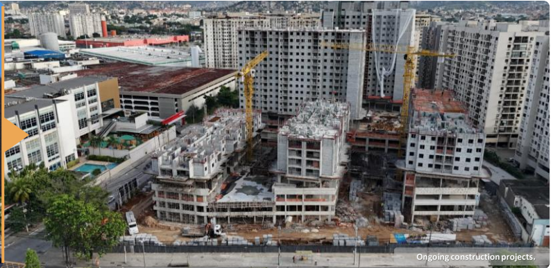
Ongoing construction projects.
